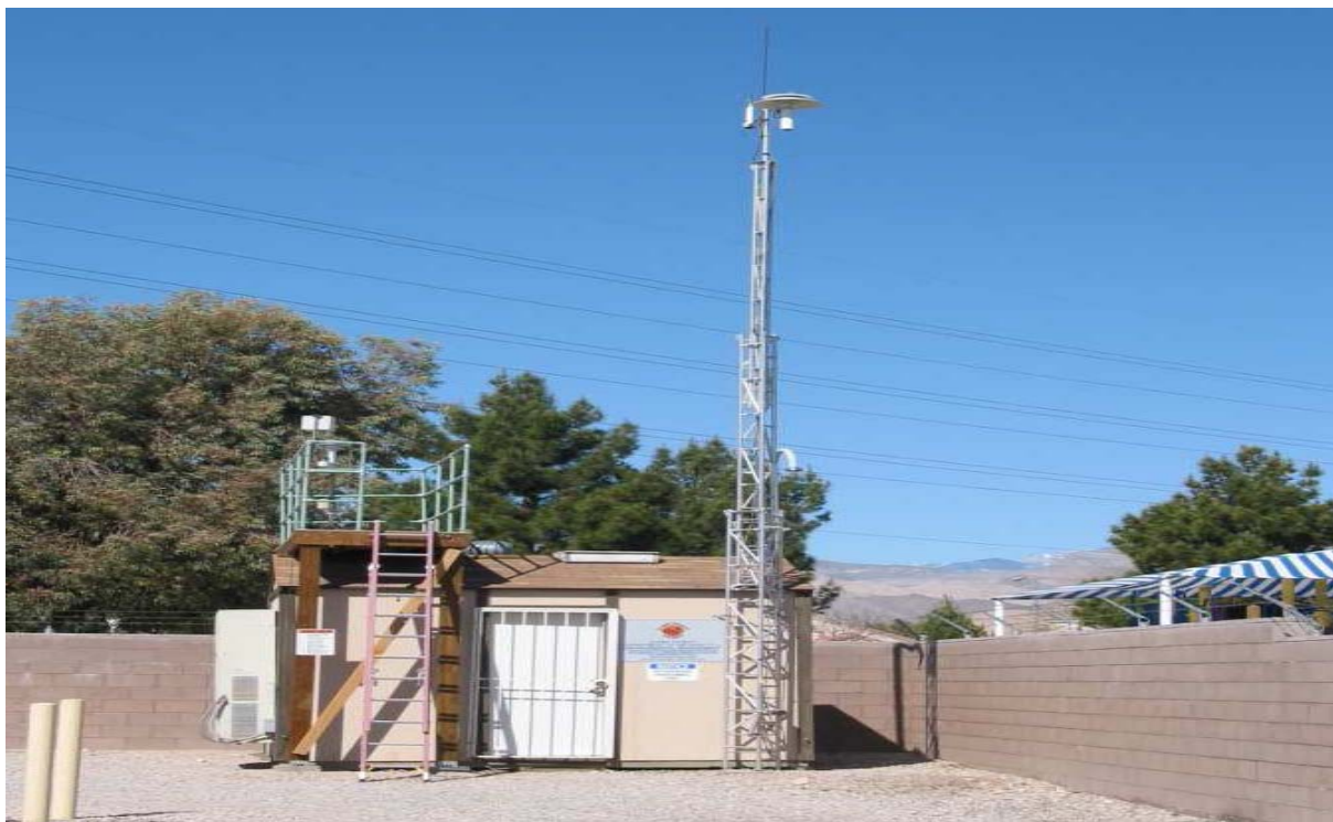
Figure 35. Lone Mountain Monitoring Station.
