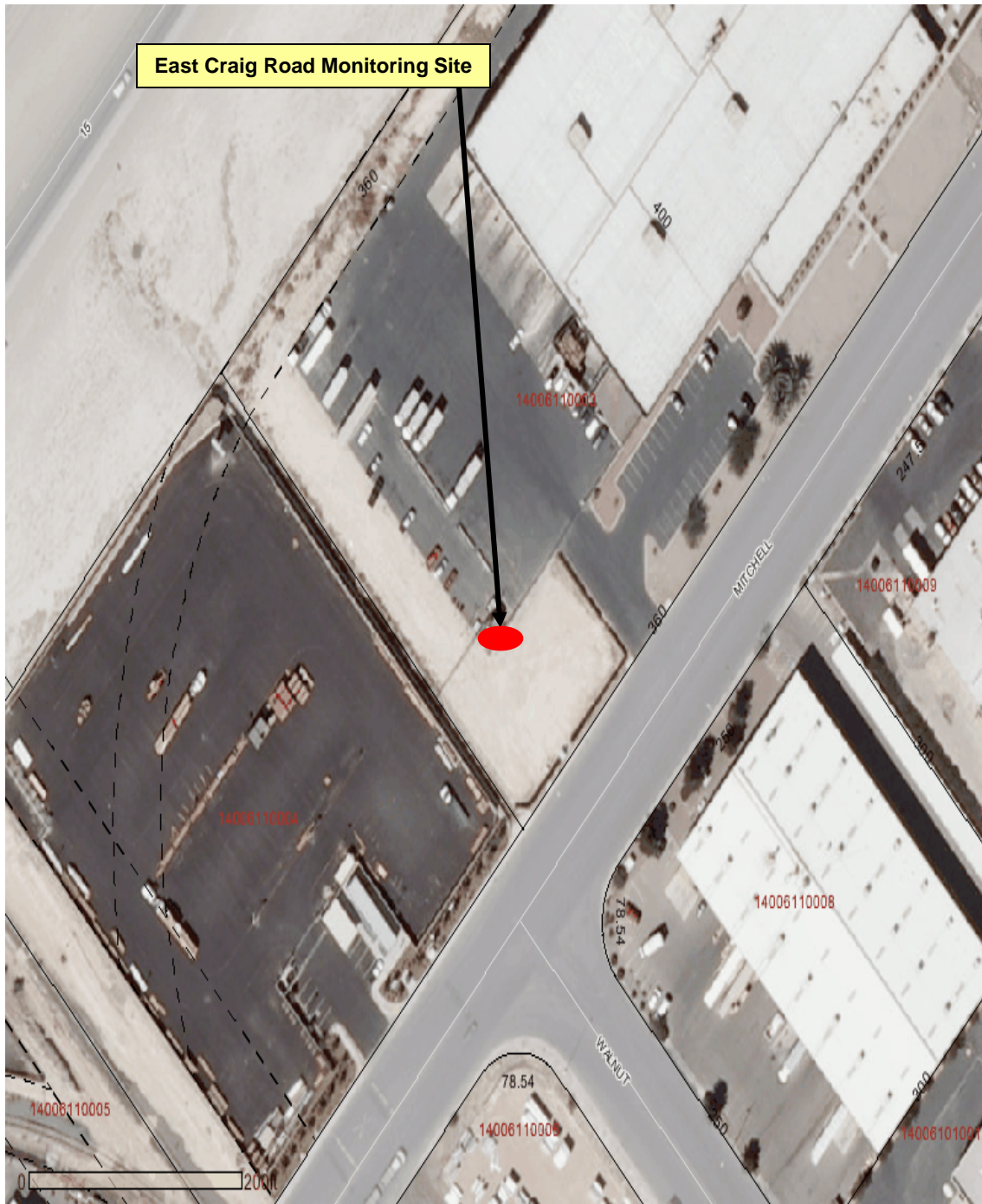
Figure 29. East Craig Road Monitoring Site, Aerial View #4.
