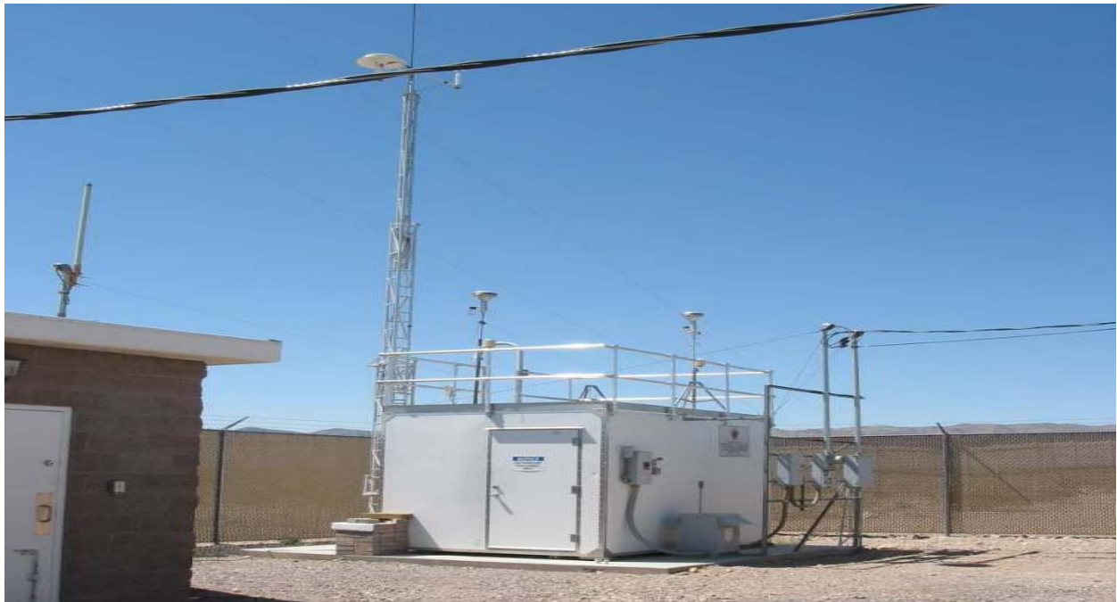
Figure 50. Jean Monitoring Site.
